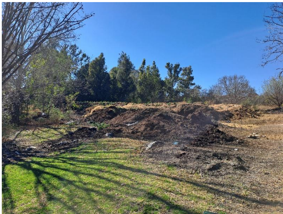
Figure 12: Soil and other rubble are dumped in the area (@Hannes Visser August 2025).
